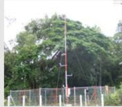
DAMU Automatic weather Station
